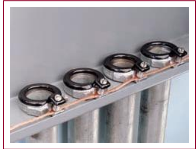
EXHIBIT 250.35 Grounding bushings used to connect a copper bonding or grounding wire to conduits. (Courtesy of Thomas & Betts Corp.)
