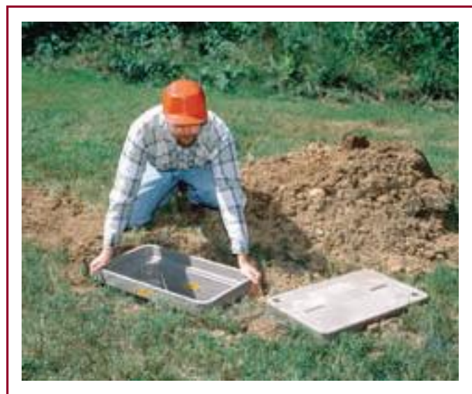
EXHIBIT 100.11 An example of a handhole enclosure. (Courtesy of Quazite/Hubbell Lenoir City, Inc.)
