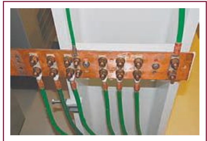
EXHIBIT 250.16 Listed connectors used to connect the common grounding electrode conductor and individual taps to a centrally located copper busbar with a minimum dimension of ¼ inch thick by 2 inches wide.
